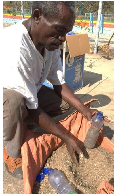
Making plastic bottle bricks At this time we packed gravel in the bottle.
